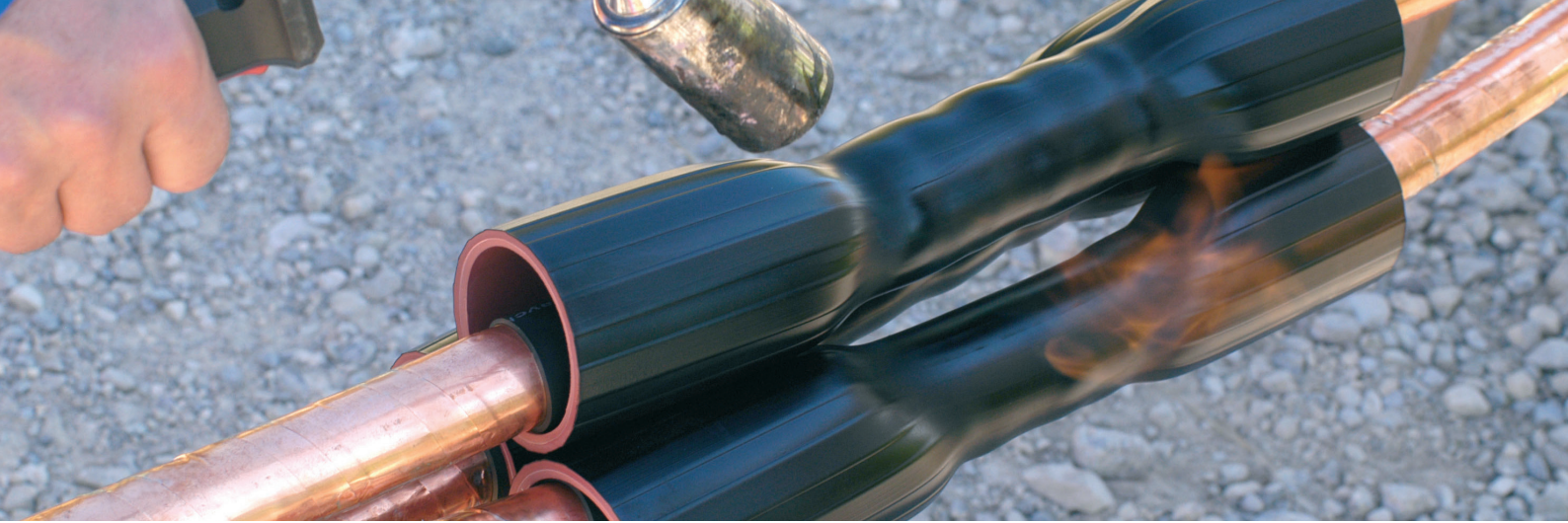
Figure Caption: Rayfit tube used in MXSU joints - Combines 3 layered, thick-wall extrusion.
